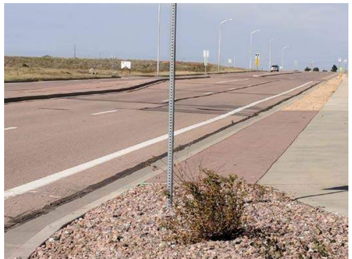
Tutt Blvd North Transition to Existing
