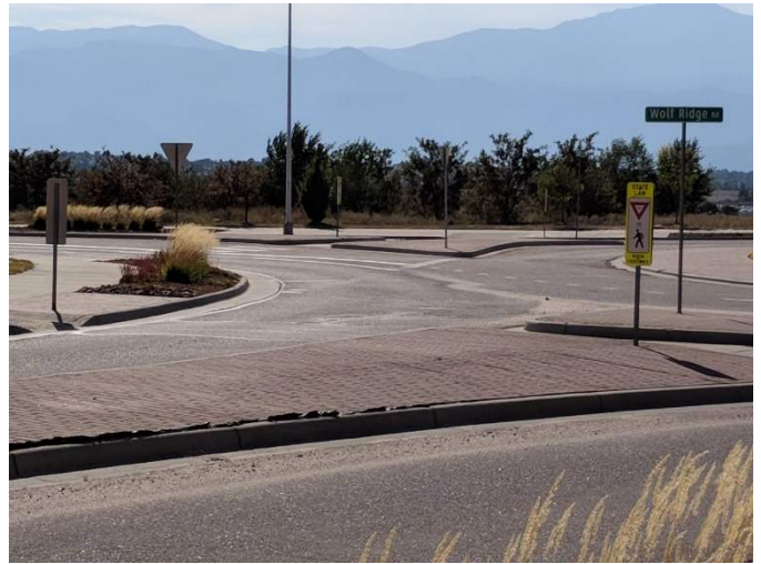
Tutt/Wolf Ridge Medians and Signage
