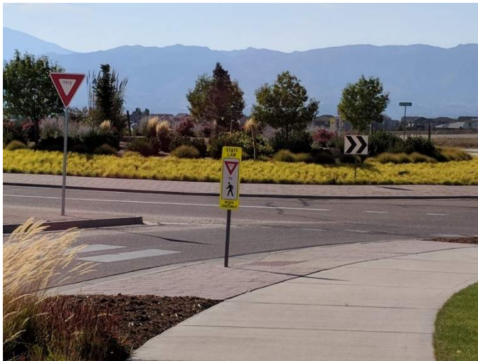
Textured Concrete and Sidewalk
