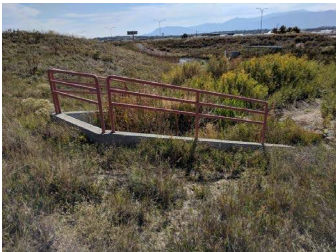
Detention Basin and Outlet
