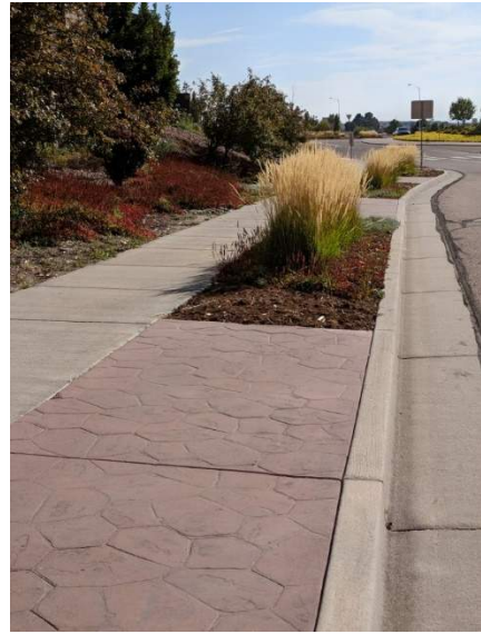
Tutt Blvd Hardscape and Curb/Gutter
