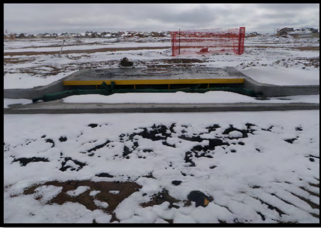
Storm inlet at Dublin Blvd.
