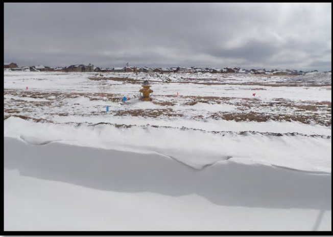
Fire hydrant in Dublin Blvd.
