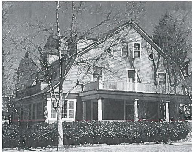
Figure 26: A wide variety of Victorian-era and early 20th century architectural styles define the neighborhood character of the Old North End.
