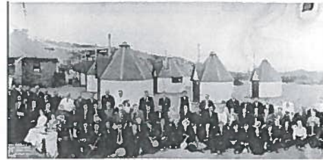
Figure 14: Octagonal-shaped tuberculosis huts, also known as "tent cottages" were designed for ample ventilation.
