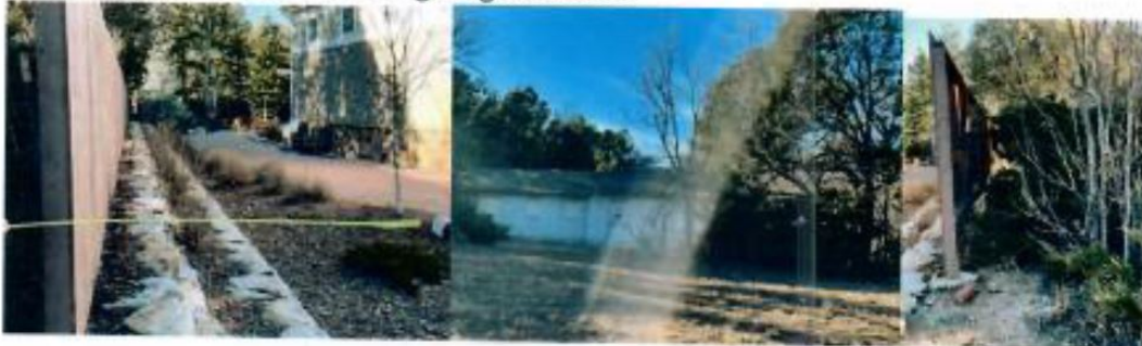
28 Marland's Retaining wall to hide abandoned house.
