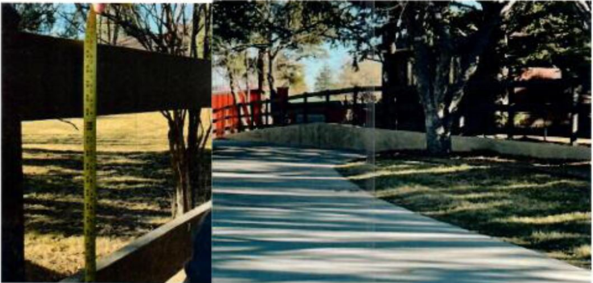
Retaining wall/fence between 29 and 35 Marland
