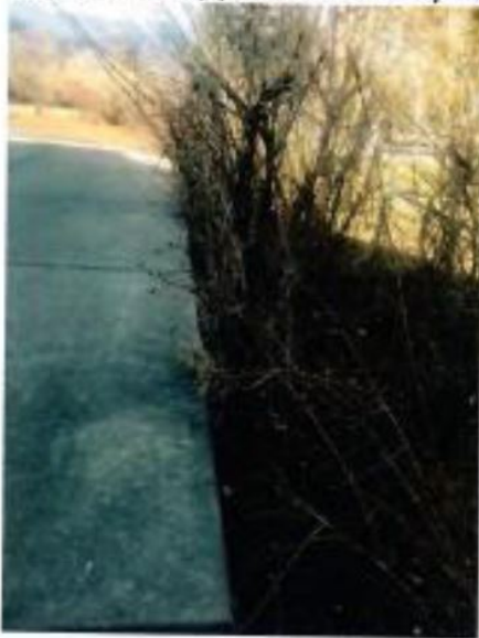
Driveway and easement between 17 and 15 Marland similar to concrete driveway of 21 Marland prior to retaining wall added in October 2018
