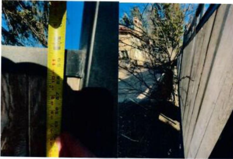
5 Marland's retaining wall
