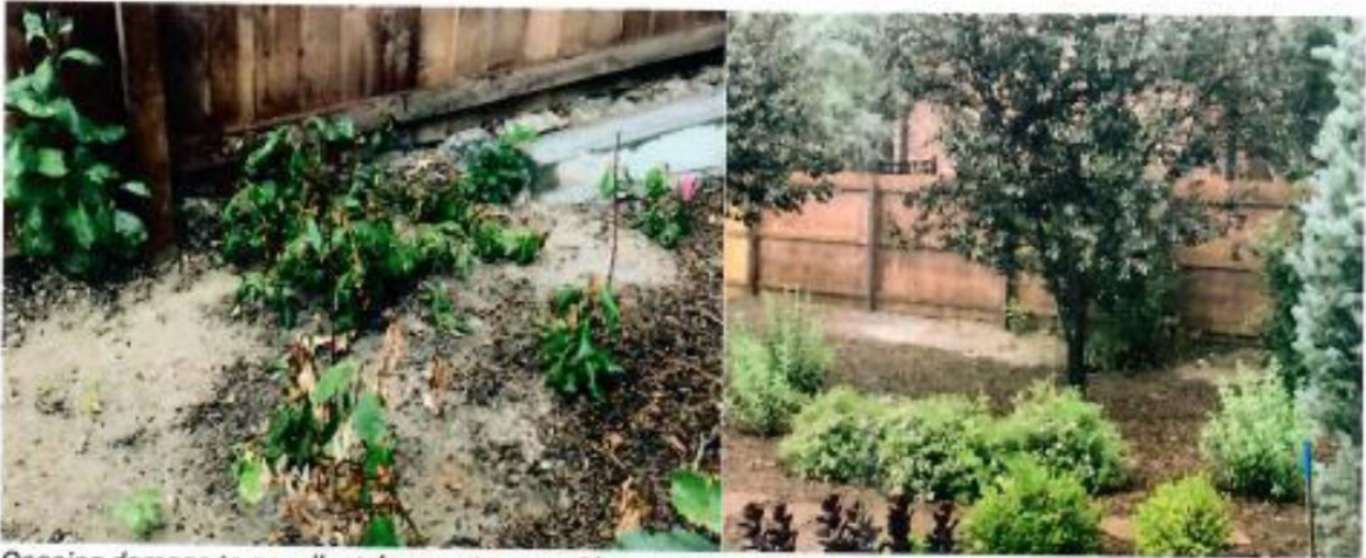
Ongoing damage to appellants' property caused by retaining wall
