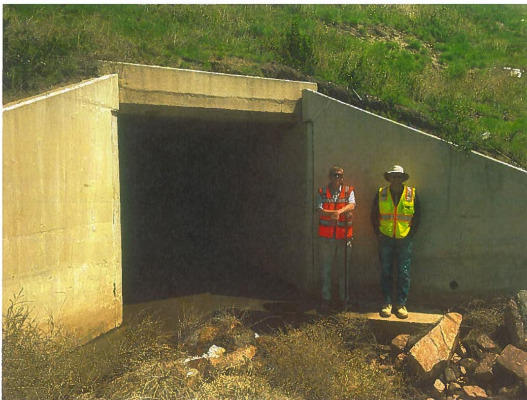
Figure 5 (Station 1+00): 8-foot by 8-foot box culvert under Powers Blvd (looking upstream)
