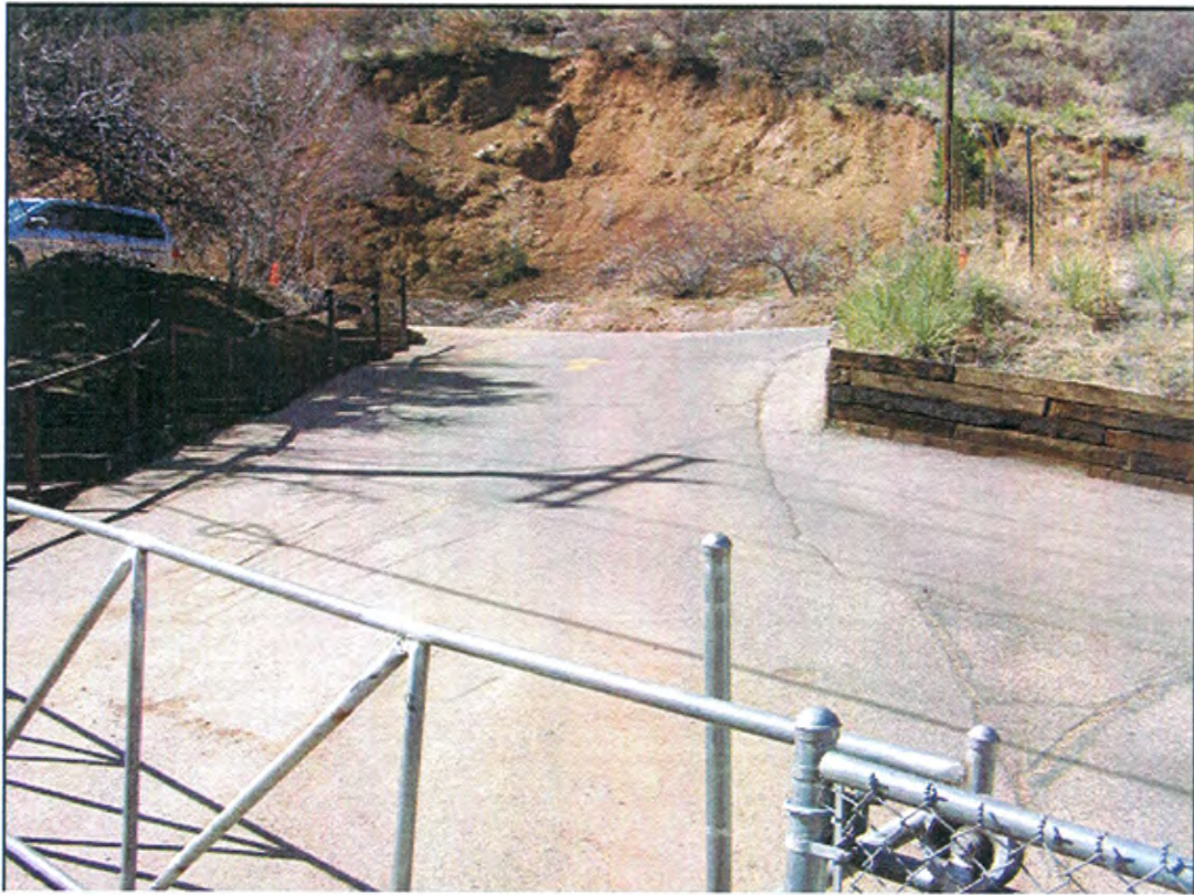
Entrance to Lot from Ruxton Ave.
