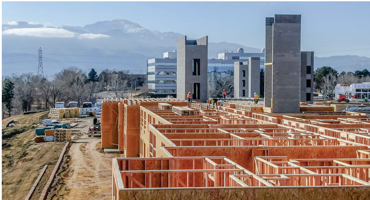
Construction taking place on an affordable housing development in 2022.
