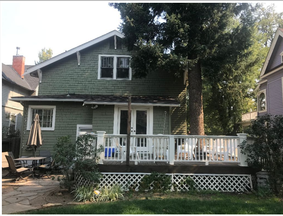
Existing rear facade with 1997 second story addition and 1991 deck addition.
