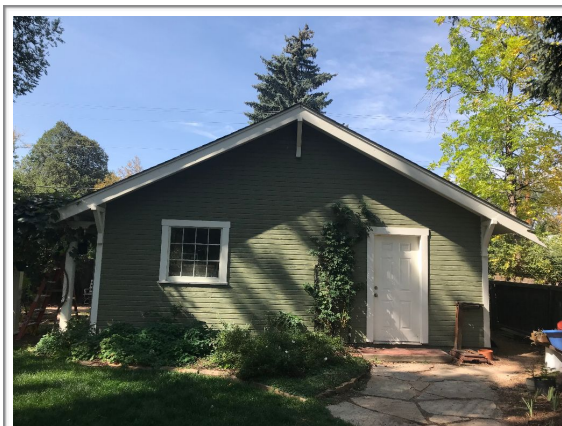
Existing 1990 garage addition located on back northwest corner of property.
