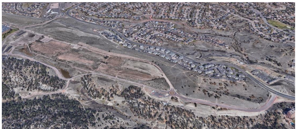
Figure 5. Poor Vehicular Access
