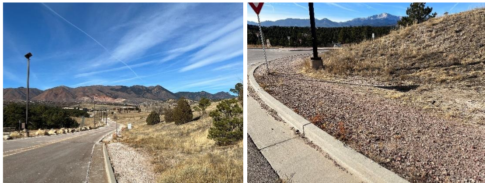
Figure 4. Poor Provision of Street Improvements for Pedestrians
