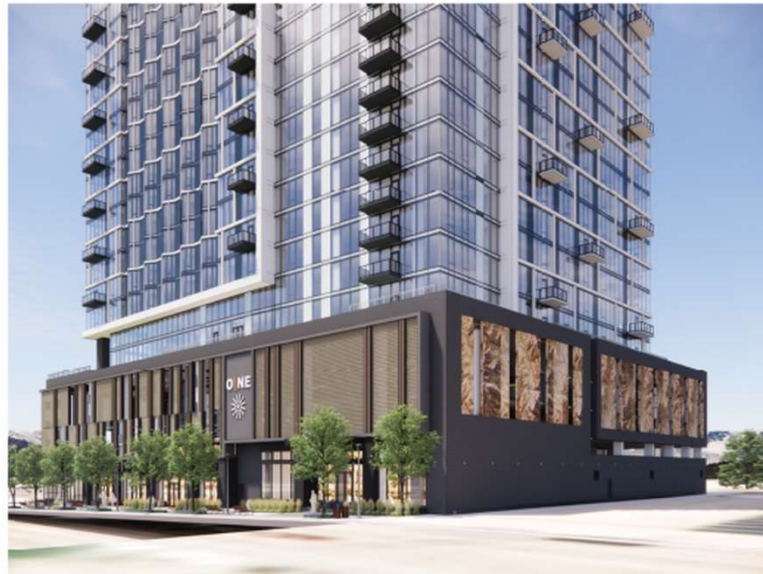
VIEW FROM SOUTHEAST CORNER
