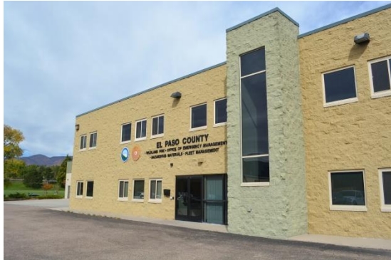
Front of EPC OEM Building
