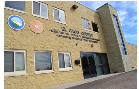
Front of EPC OEM Building
