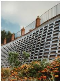
GRAVITY TYPE WALL
