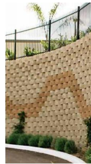
REINFORCED EARTH TYPE WALL
