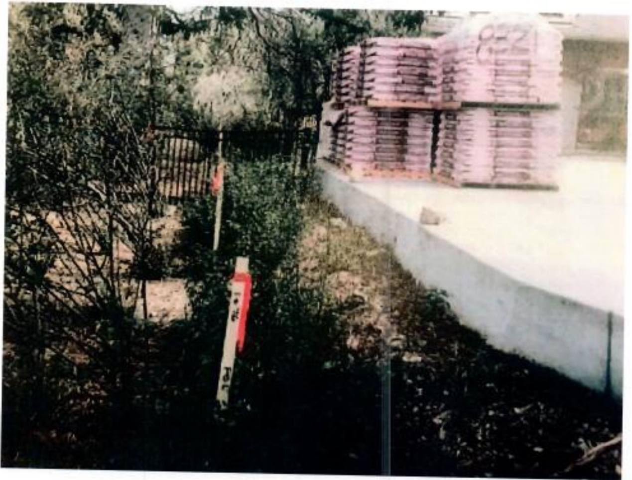
Photo A: Topography Before Retaining Wall
