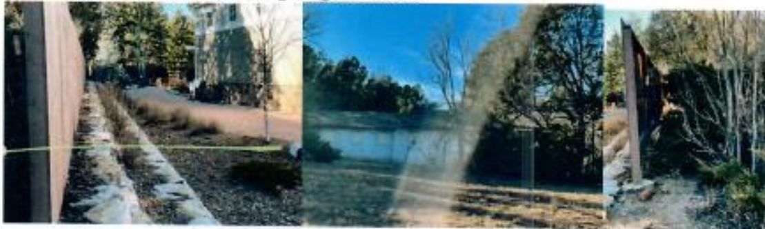
28 Marland's Retaining wall to hide abandoned house.
