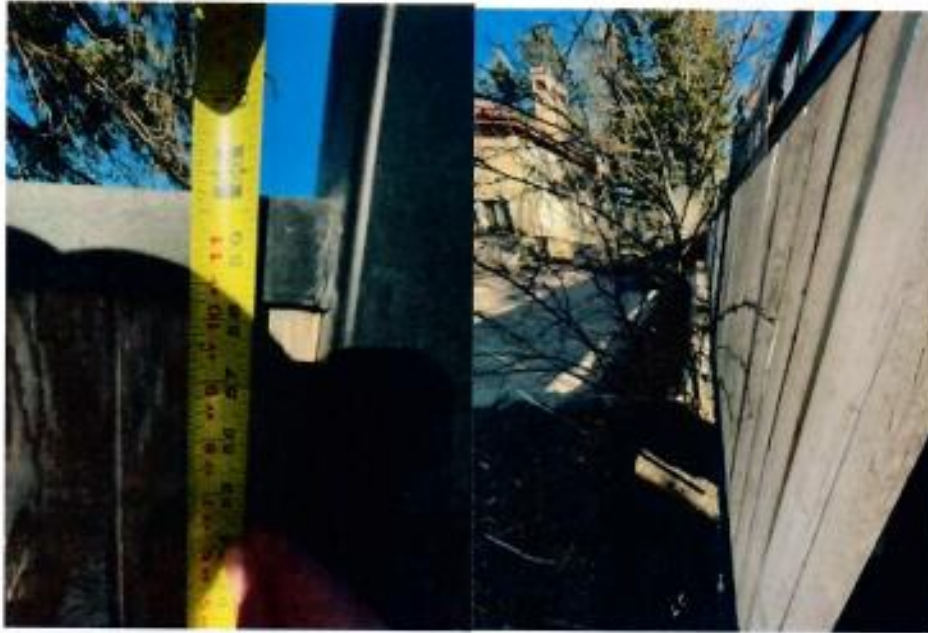
5 Marland's retaining wall
