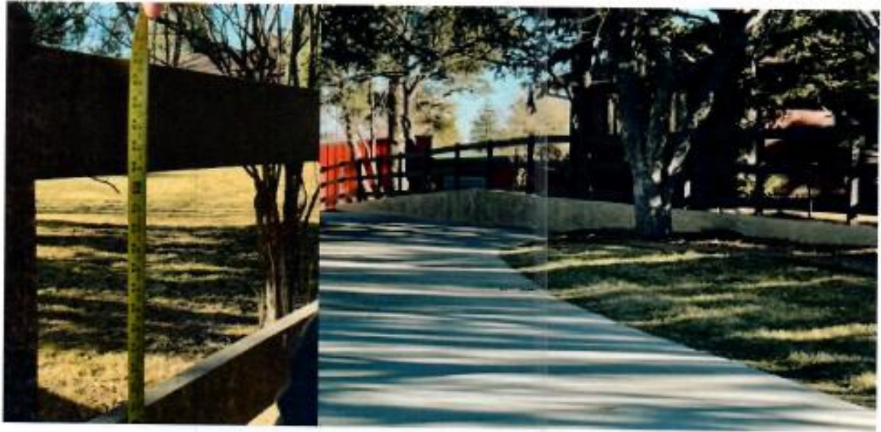
Retaining wall/fence between 29 and 35 Marland
