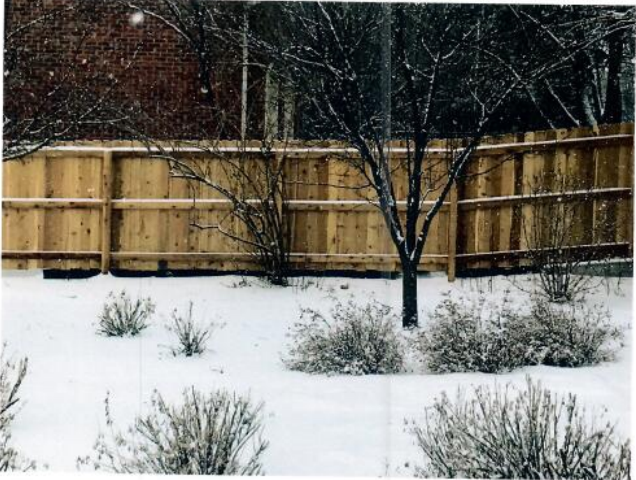
Photo C: Slope of Retaining Wall
