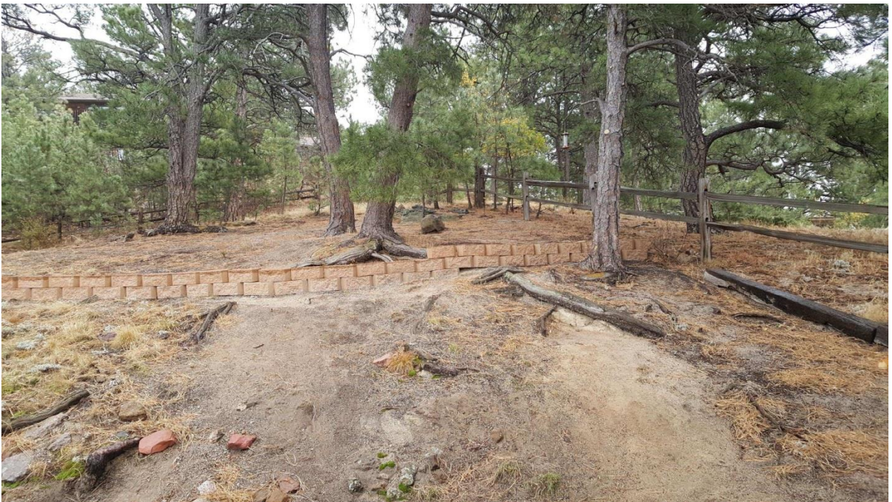
(View from the top of retaining wall next to the driveway)
