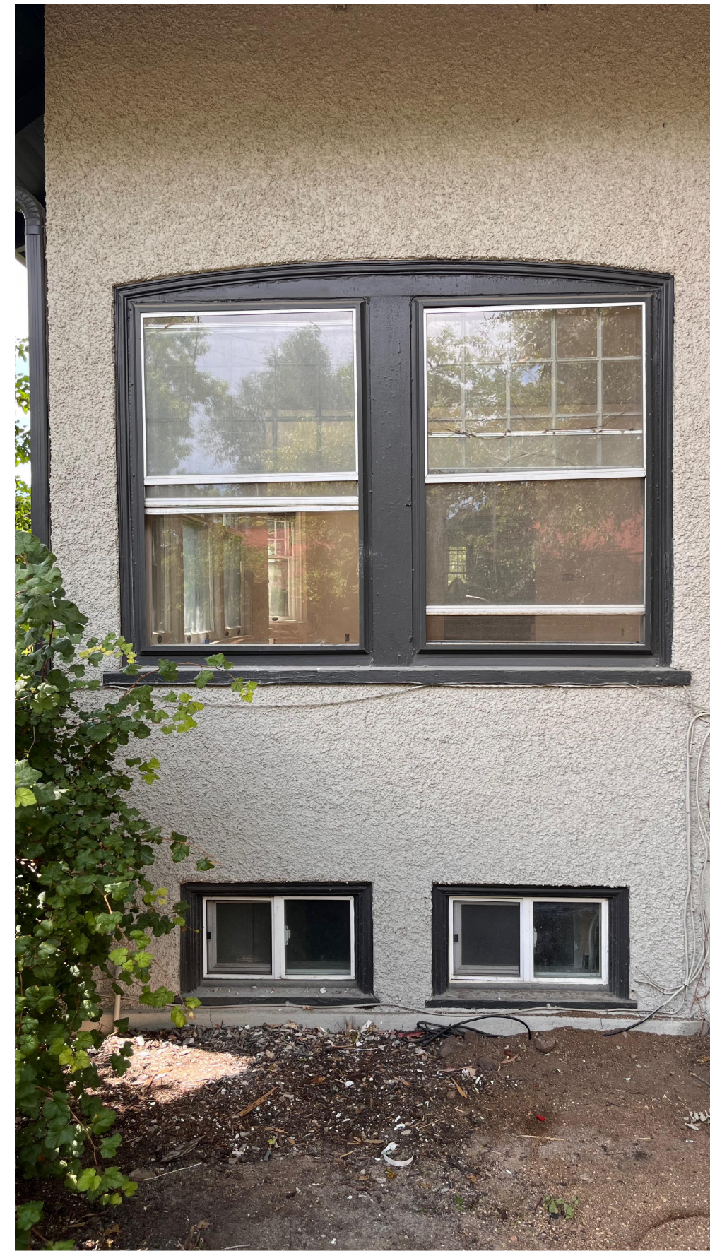
3 A-2 EXISTING EAST WINDOWS
