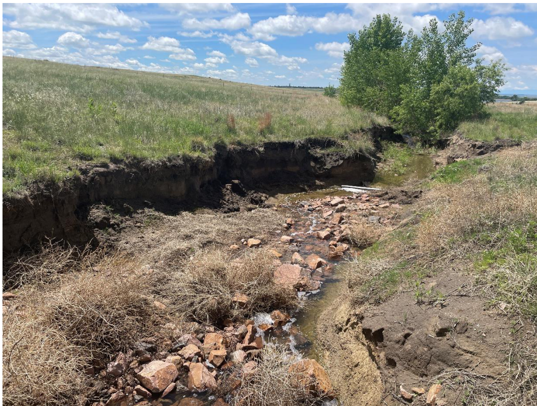
Figure 6 (Station 1+50): Degraded section downstream of culvert with rip rap rundown (looking downstream)
