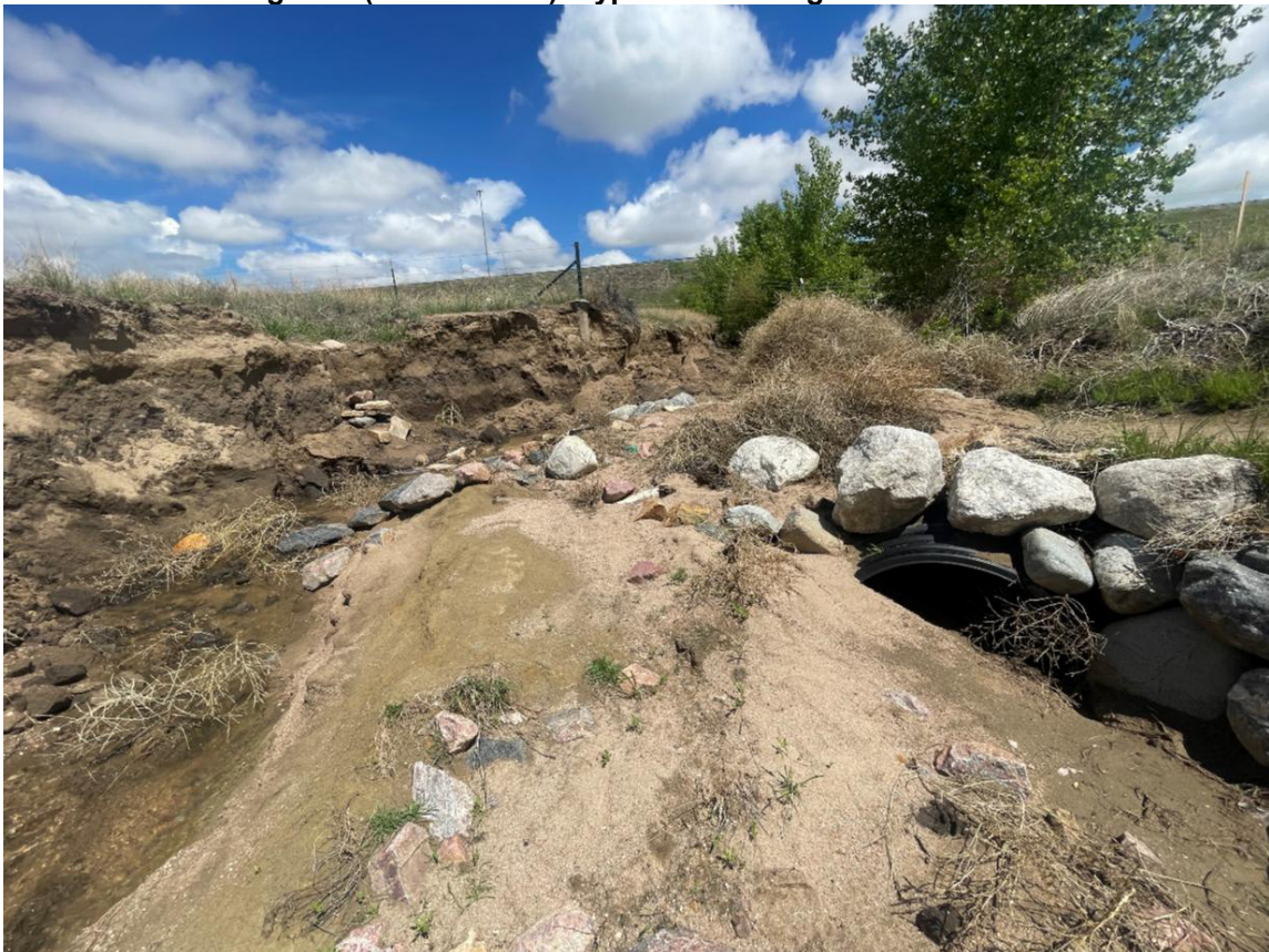
Figure 9 (Station 3+50): Flanked culvert and failed trail crossing (looking upstream)
