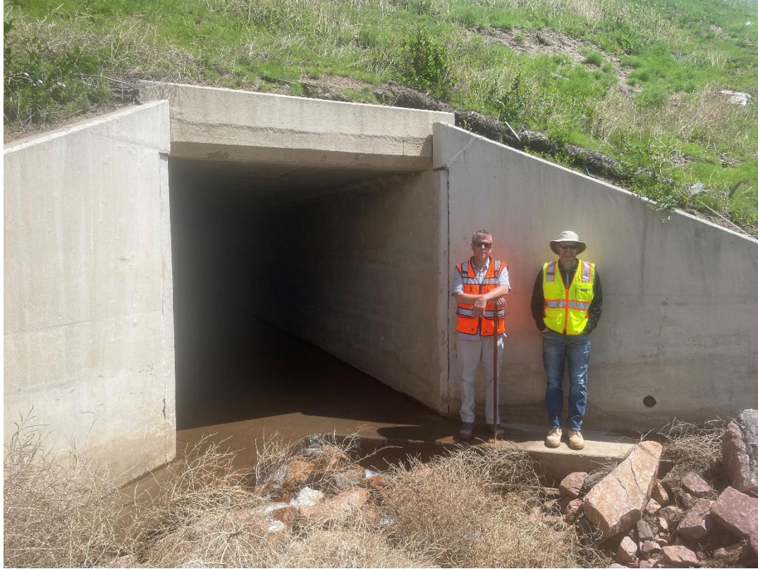
Figure 5 (Station 1+00): 8-foot by 8-foot box culvert under Powers Blvd (looking upstream)
