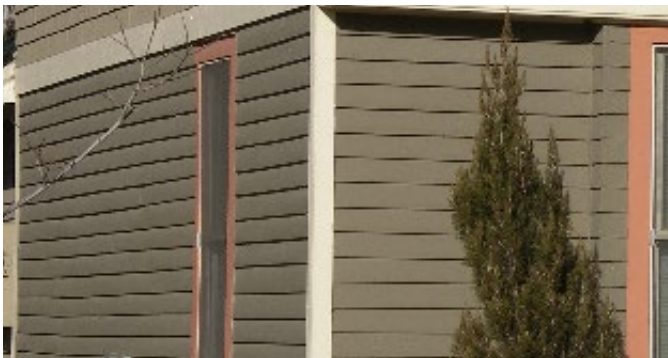
Exterior wall repaired by partial replacement of damaged bevelled cedar siding to match existing siding that has been retained and repaired.
