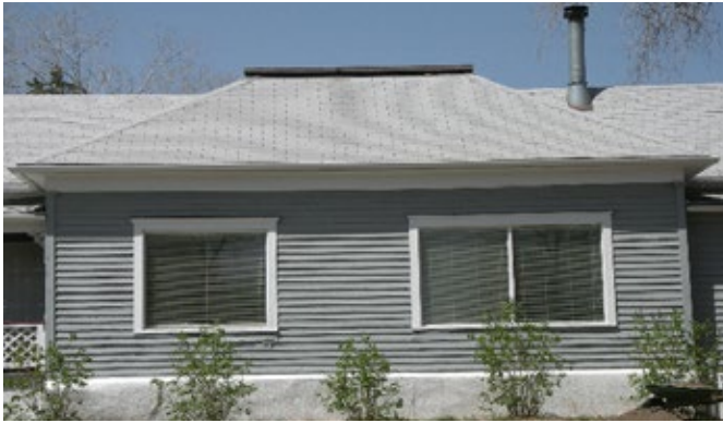
Replacement windows that do not respect original pattern of tall narrow grouped double sash windows common to the style of house.
