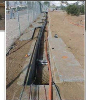
Electrical - Installed two conduit runs of 270' and electrical distribution system.
