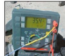
Ground system installed, tested and certified to Motorola R-56 Standards
