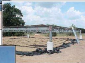
Precision Anchor Bolt Placement
