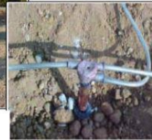
Grounding - 9 ground rods with CadWeld connections
