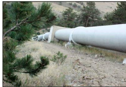
Finished Buried Conduit prior to Erosion Control
