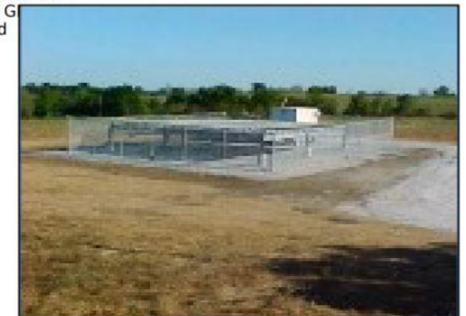
Finsihed project with road, parking lot, fence.
