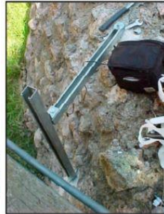
Epoxied Unistrut Conduit Supports in Solid Rock
