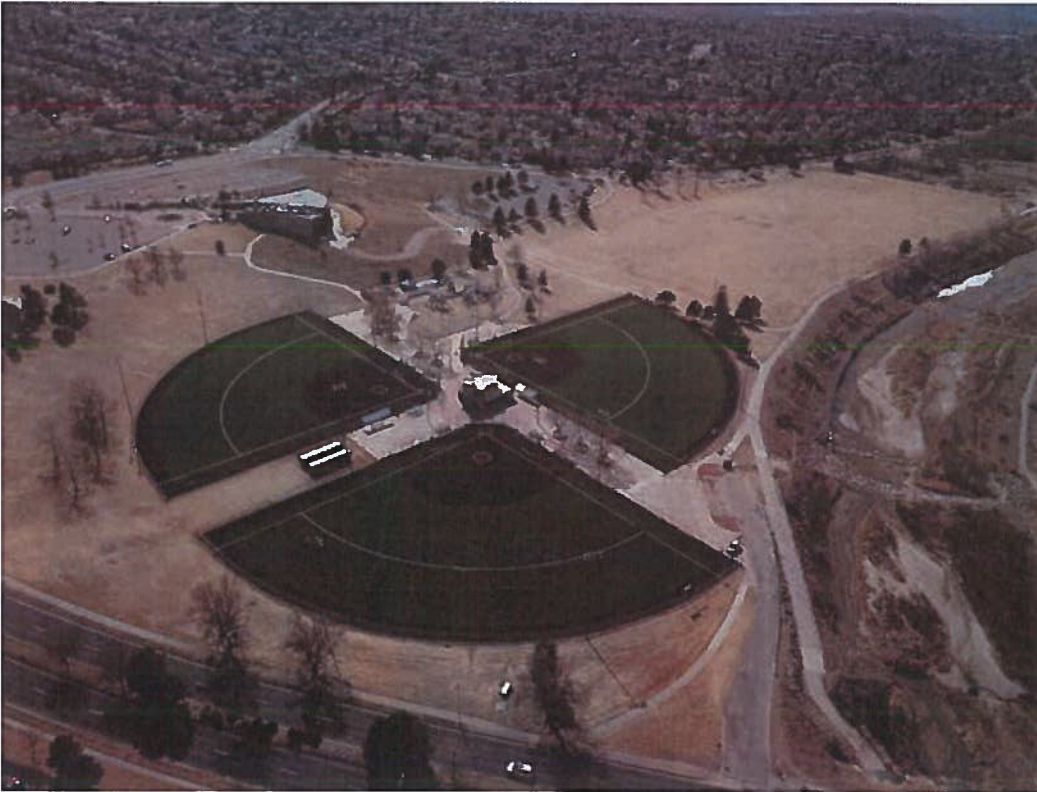
Cottonwood Creek Ballpark with the new artificial turf installed.
