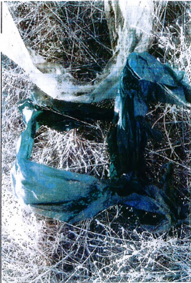
Photograph 18 - Looking at large amounts of plastic that were pulled out of Boring S2-3 during drilling.
