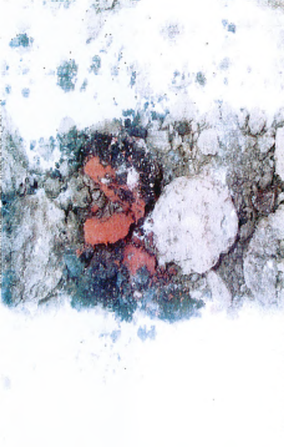
Photograph 12 - Looking at wood and brick fragments that were collected in Boring S2-1.
