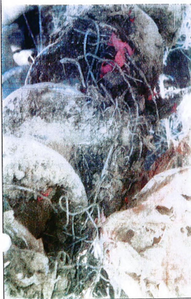
Photograph 17 - Looking at a large amount of galvanized wire that was wrapped around the augers in Boring S2-3.
