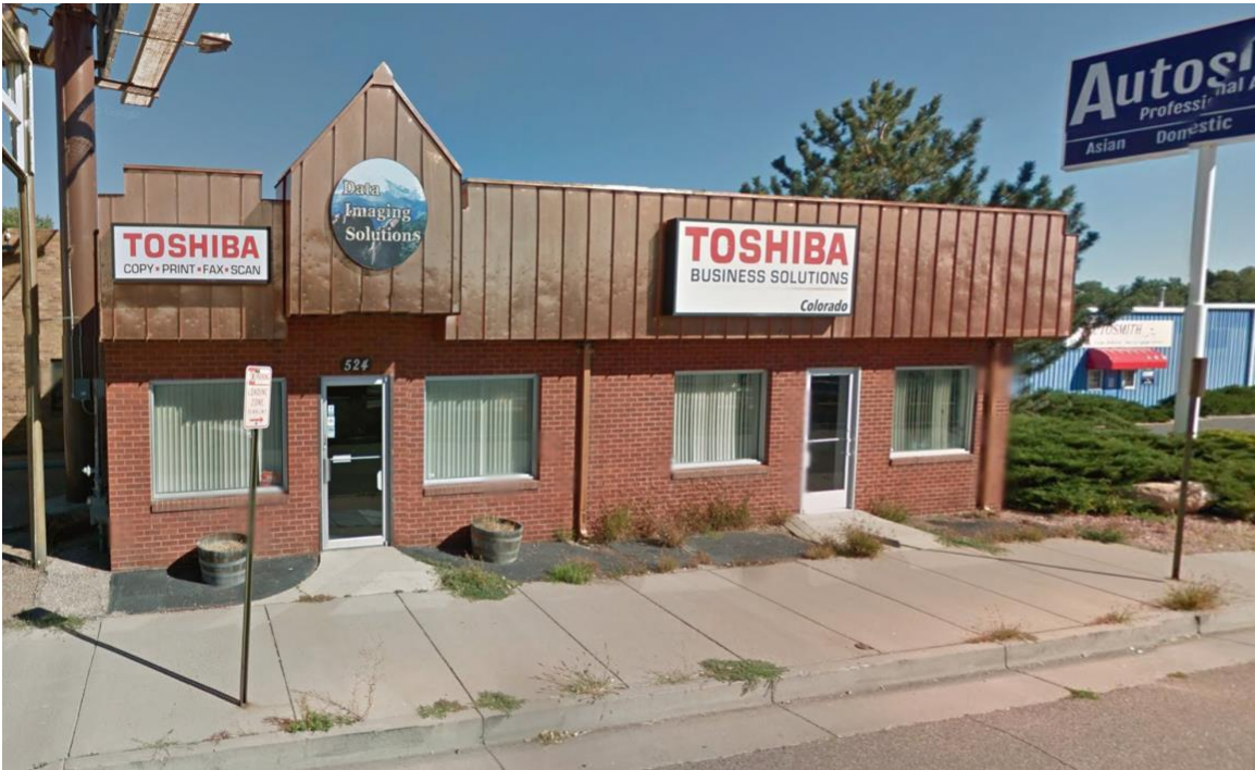
Existing Building from Pikes Peak Ave. South elevation
