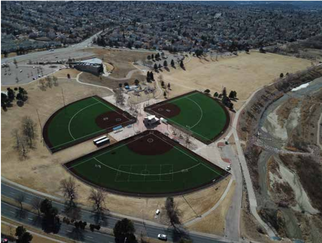
Cottonwood Creek Ballpark with the new artificial turf installed.
