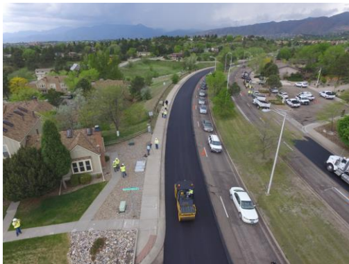
Rockrimmon Blvd. Paving
