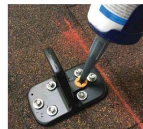
Insert tip of UNIRAC approved sealant into port and inject until sealant exits vent. Continue array installation, attaching rails to mounts with provided T-bolts.
