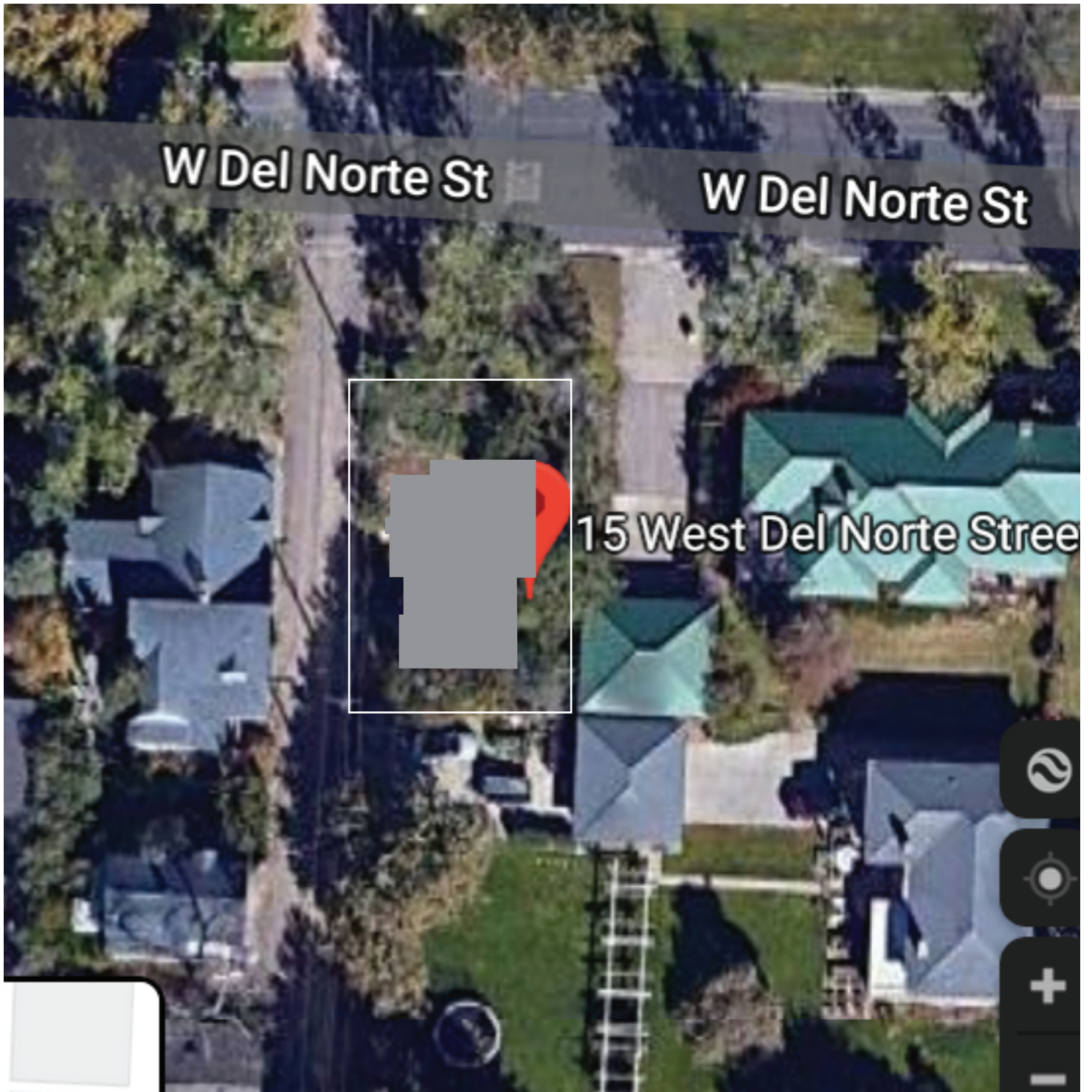
General location of structures on properties adjacent to 15 W Del Norte
