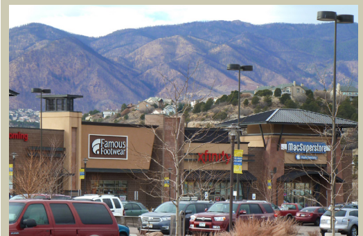
Figure 5.2-A. Example Photos of Existing Exterior Materials
