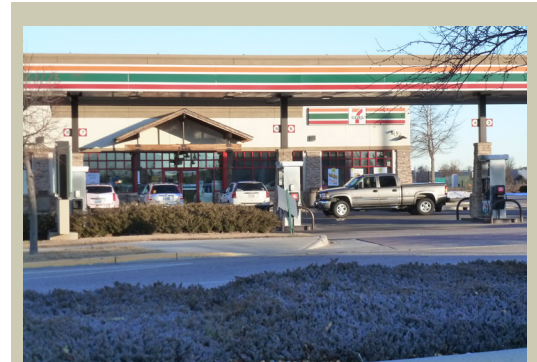
Figure 6.6-A. Example Photo of Convenience Store / Gas Station Canopy
