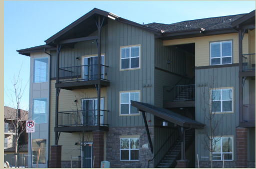
Figure 6.7-B. Varied Multifamily Building Materials
