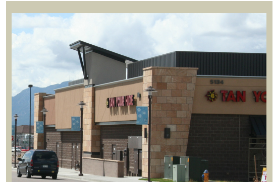
Figure 5.7-A. Example Photo of Rooftop Screening
