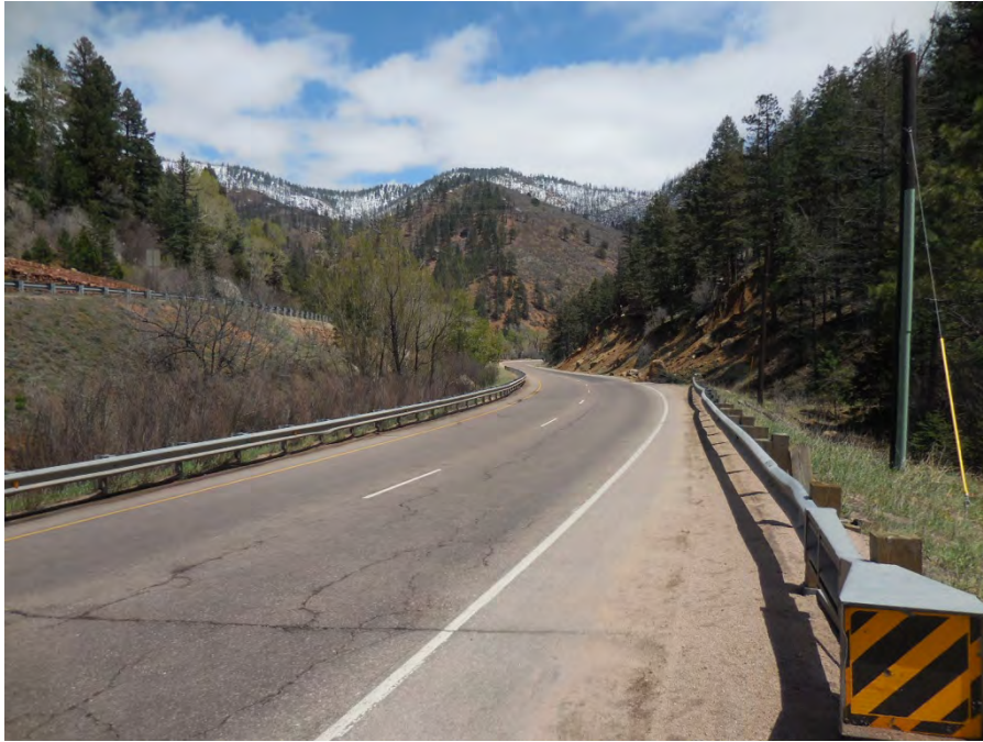
Highway 24 looking northeast along east-bound lanes. Subject property is to right.
