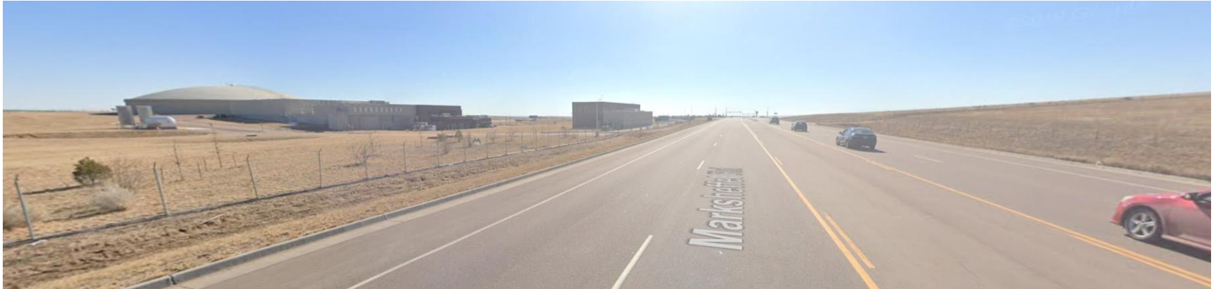
LOOKING SOUTH ALONG MARKSHEFFEL - CITY WATER FACILITY ON LEFT
