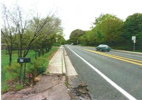
Looking South Along Cresta Road
