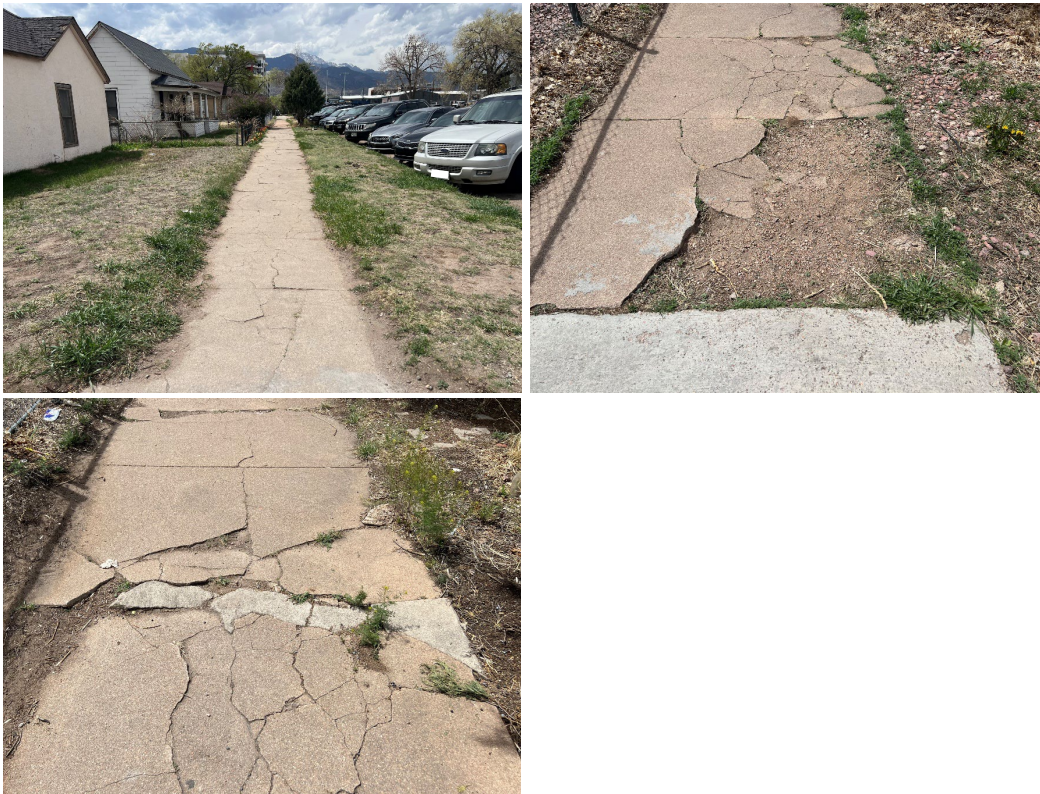
Figure 6. Cracked and Uneven Surfaces for Pedestrians
