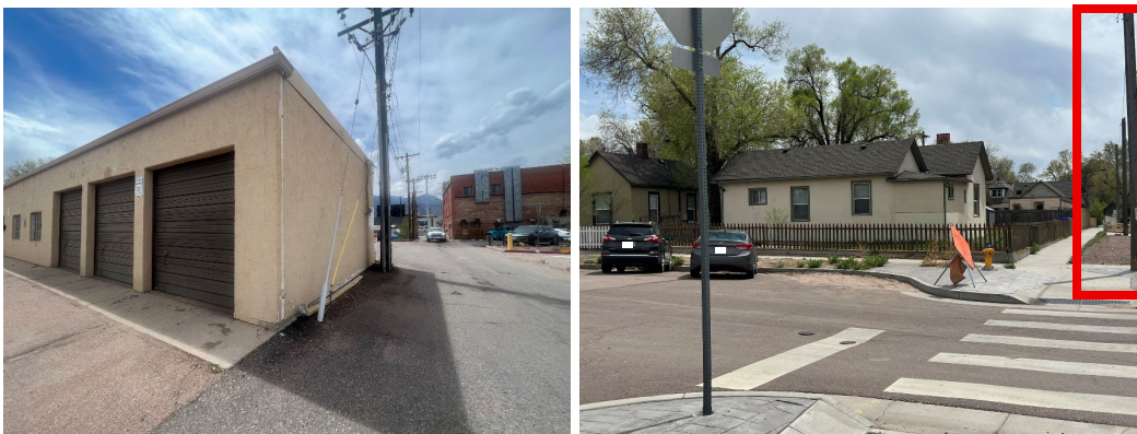
Figure 13. Presence of Overhead Utilities
