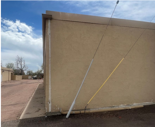
Figure 3. Deteriorated Gutters/Downspouts
