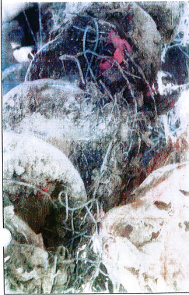
Photograph 17 - Looking at a large amount of galvanized wire that was wrapped around the augers in Boring S2-3.
